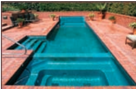
Klaser Tile uses conventional mortar bed and butter-mix methods to achieve the perfect substrate – this takes tremendous care in floating the mud bed to strict industry standards to get the correct radius dimensions for domes and pools.
